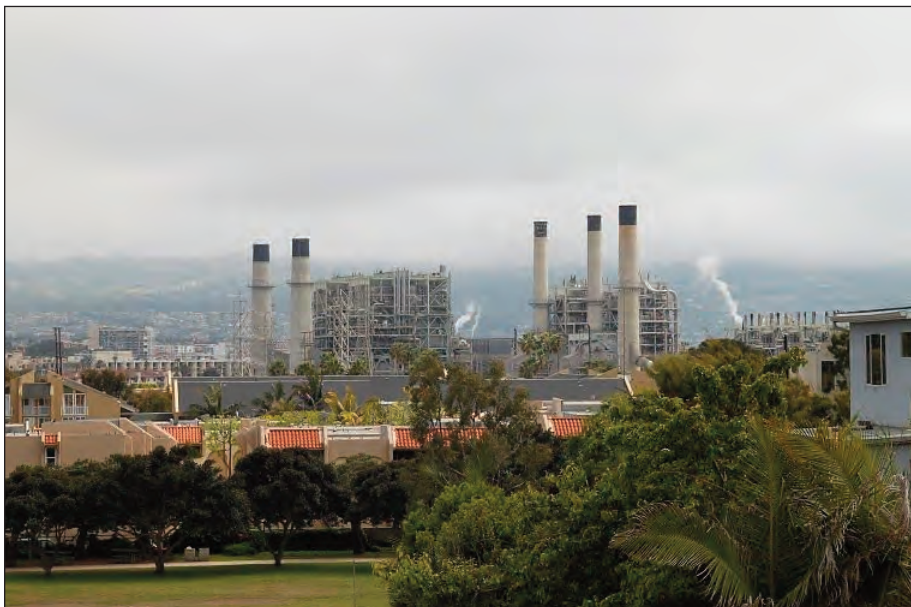
AES Redondo Beach Power Plant.
